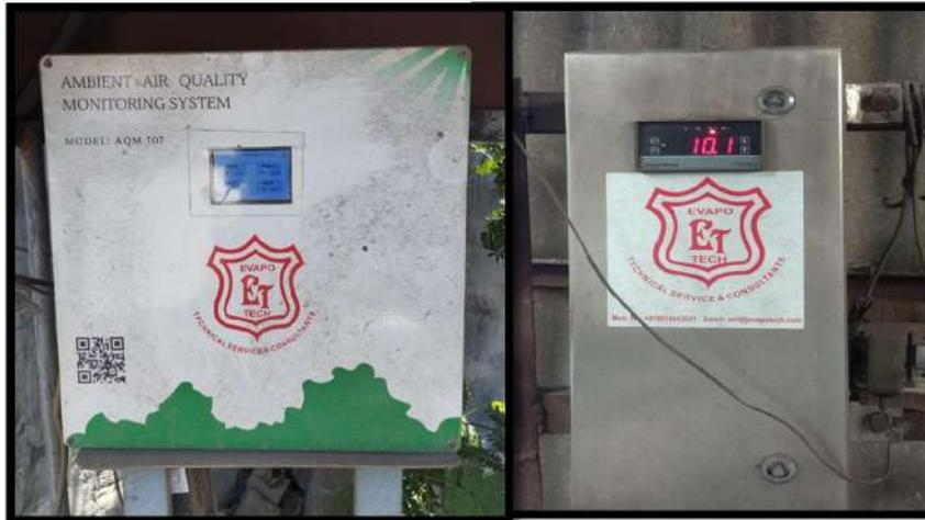
Photographs showing AAQMS & OCEMS installed
